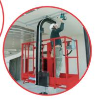
Activated directly from the platform with a push of a button, the sheet travels up the track into the overhead position, then retaining the drywall sheet in the proper location, leaving the worker free to screw or nail it to the joists/studs.
